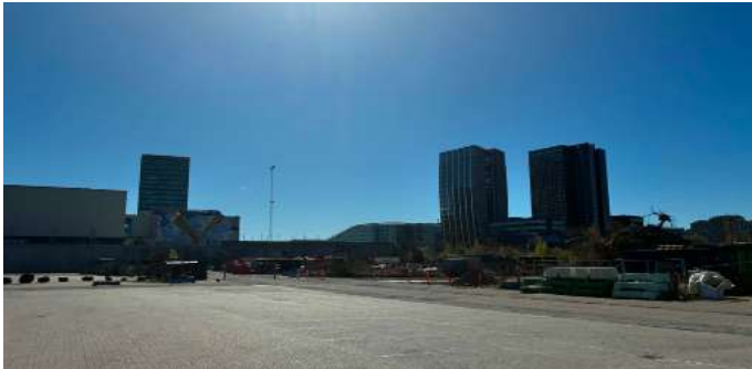
Illu. 18 Site viewed from west
