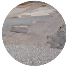
Many asphalt layers
