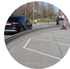
Temporary traffic barrier
