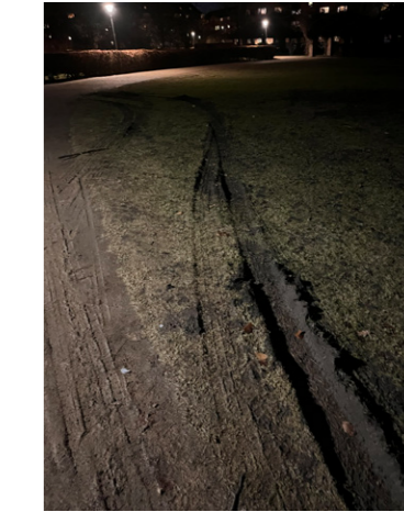
Fig.33 Photo of eroded main path surface under night conditions.
