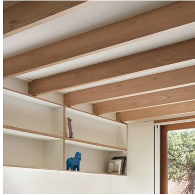
Plaster walls and ceiling Pine beams and columns
