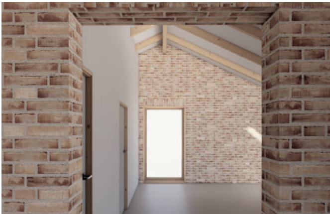
Figure 140. Gable window, brick jack arch
