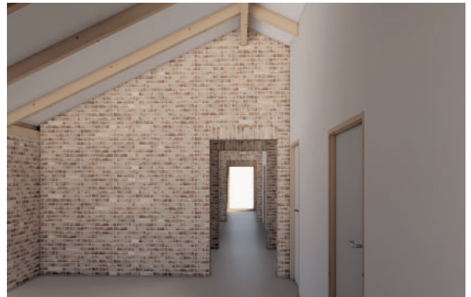
Figure 139. Opening, brick jack arch
