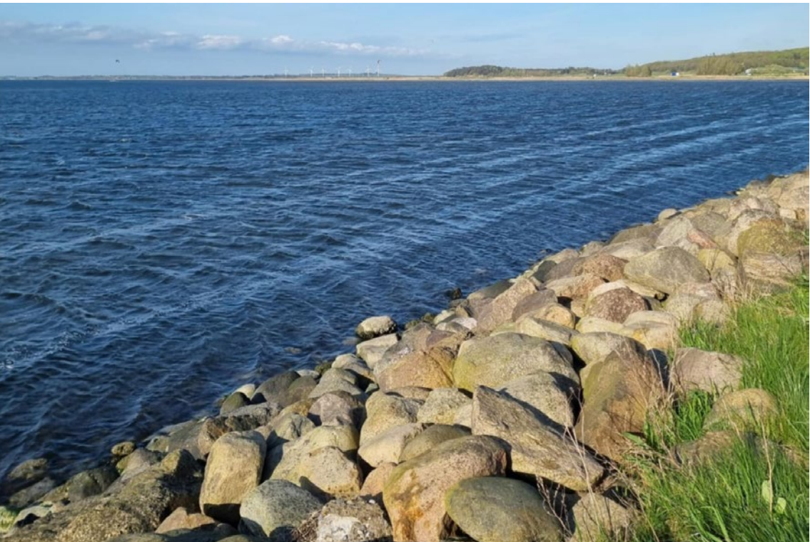
ill. 57. Hybrid structure erosion control, Nibe
