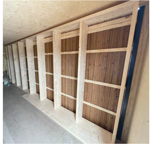
Figure 4.2. Interior view of the ventilated facade, without any wall elements.
