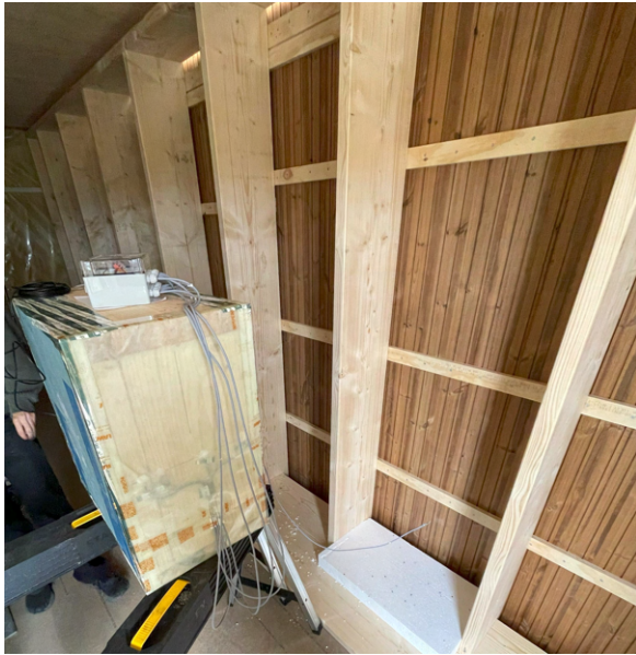
Figure A.10. Installing of the sensor in the ventilated cavity.
