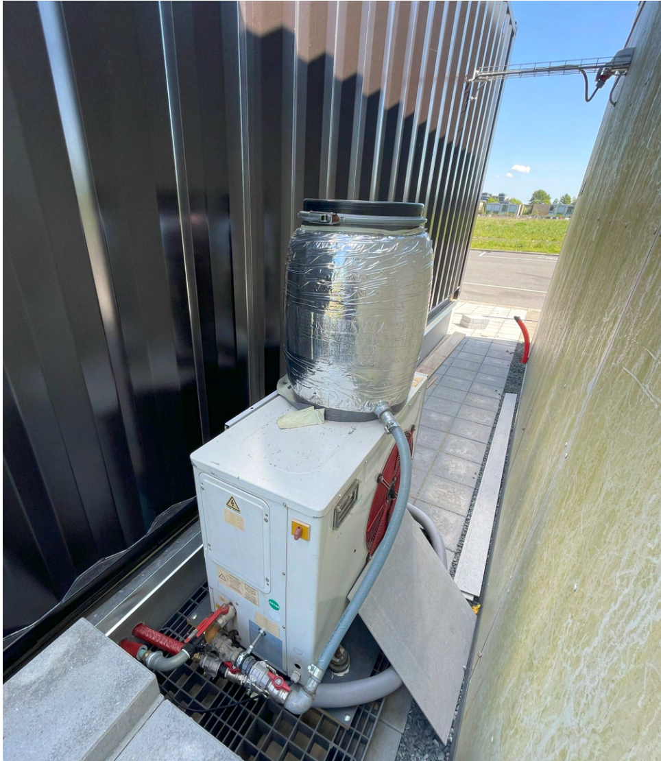
Figure A.18. Air to water heat pump, that delivers the cold water continuously to the buffer tank.
