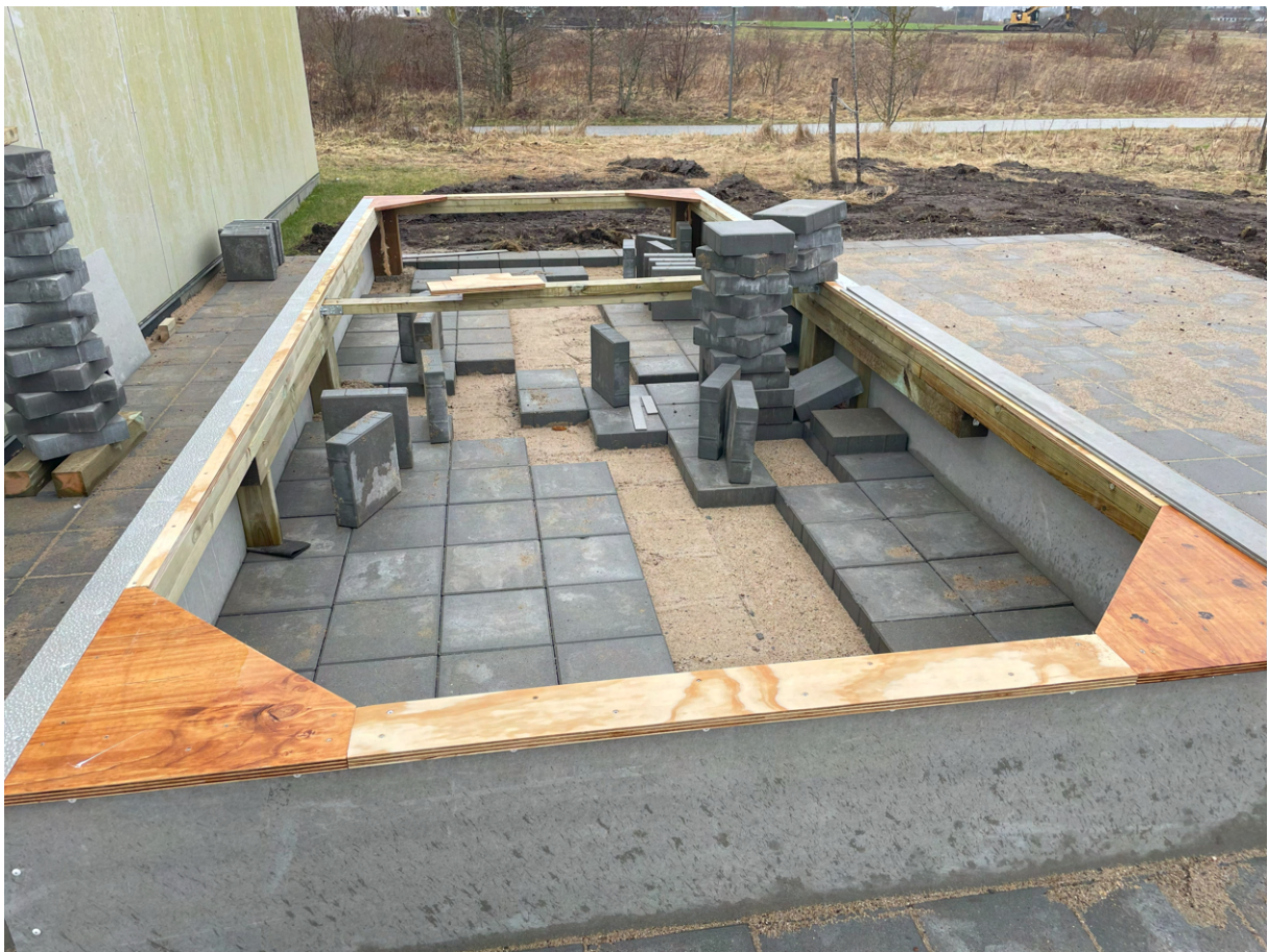
Figure A.20. Photograph of the raised foundation for the container and the inclosed crawl space.
