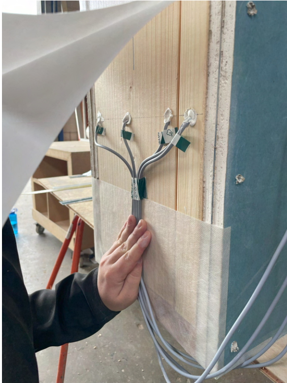
Figure C.23. Mounting of sealing tape, for the sides of the element. It shows how the cable holes is filled with sealant to make it air tight.
