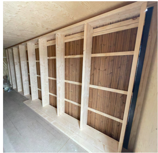
Figure A.6. Interior view of the ventilated facade, without any wall elements.
