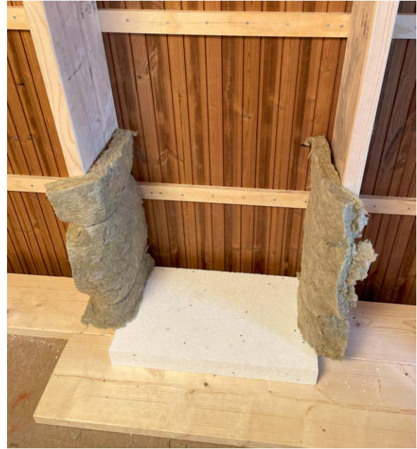
Figure A.11. Side insulation is mounted, so a wall element can be lifted into place.
