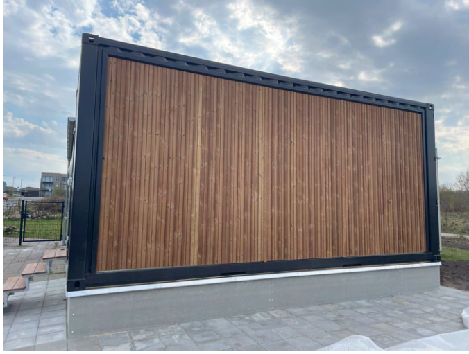
Figure 4.1. Outside view of the facade facing north, with the rain screen for the wall elements.
