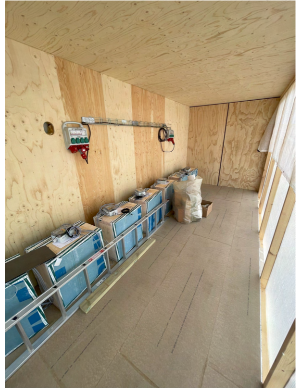
Figure B.2. The inside of the container with added insulation on the floor, and storage of the wall elements.
