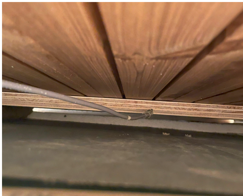
Figure C.19. Sensor placement inside ventilated cavity
