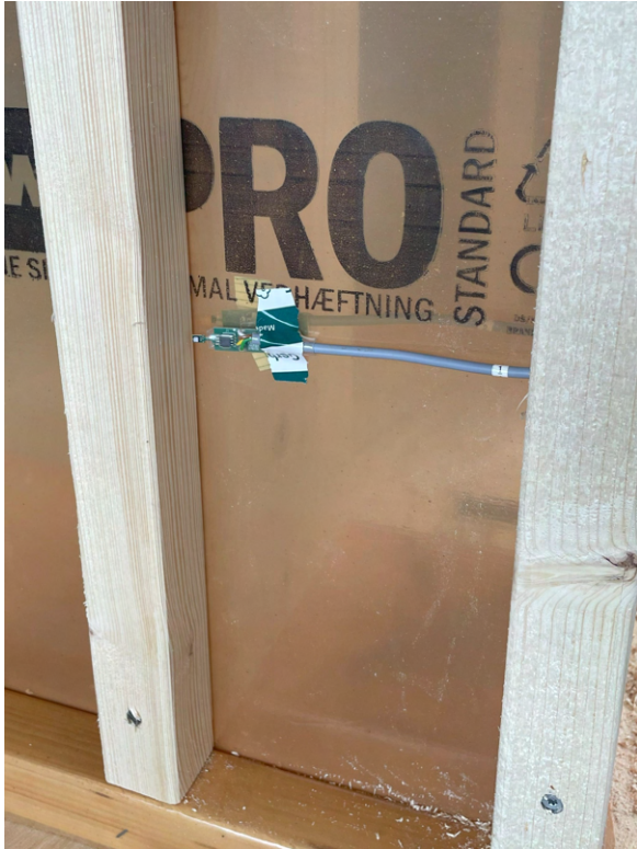
Figure C.14. Photo showing the sensors placed before and after the water vapour barrier.
