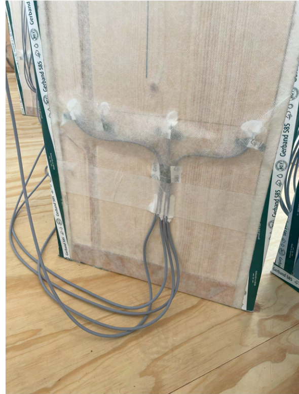
Figure C.24. After mounting sealing tape on the sides, additional sealant was used to close the cable penetration at the overlap between the two vapour barrier sheets.
