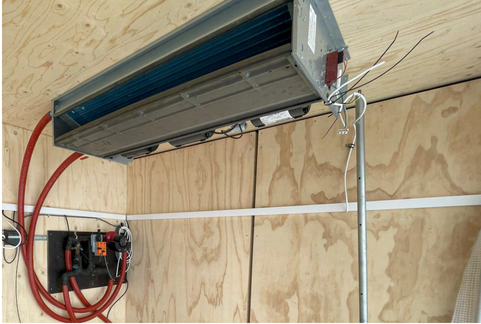
Figure A.17. The cooling system, with the mixing loop mounted on the wall. The cooling power is adjusted with the motorized three-way valve.
