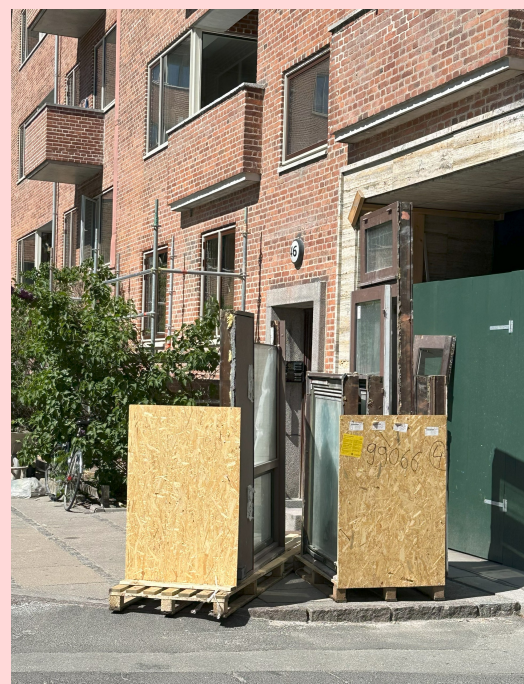
Image 6.10. Dismantled windows stored on pallets, waiting until enough have accumulated for efficient collection and transport, (Own photo)
