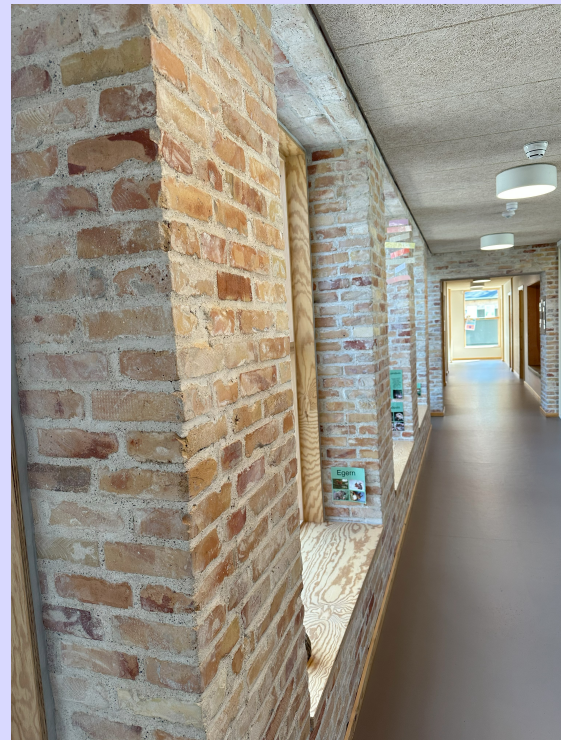
Image 6.7. The indoor wall with reused bricks (Own photo).
