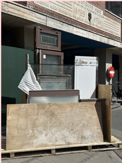
Image 6.10. Dismantled windows stored on pallets, waiting until enough have accumulated for efficient collection and transport, (Own photo)
