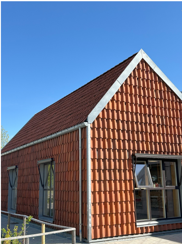
Image 7.1. Roof tiles that now also function as facade cladding, (Own photo).
