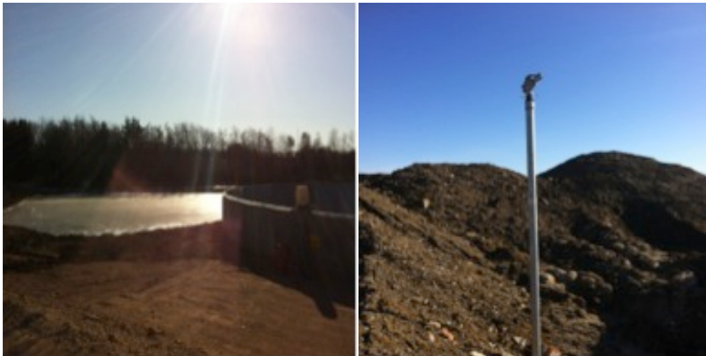
Photo 7 Water system. the water is transported via pipes to the basin and will be cleaned with filter from oil and polluting substances. Afterwards the water runs into the artificial lake.
