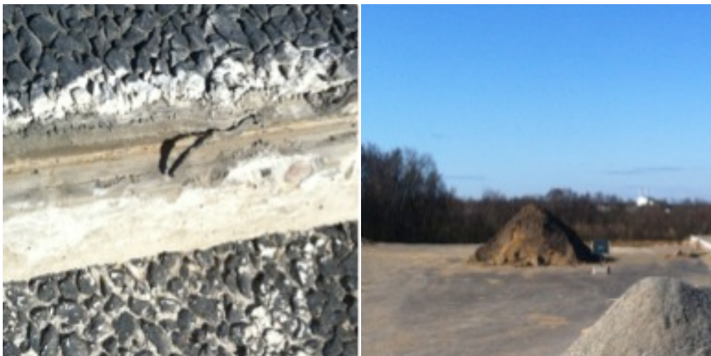
Photo 9 Concrete plates from Aalborg Politigården polluted with PCB. 5cm of concrete need to be taken of and send to destruction in order to use the rest of the concrete plate (left).
