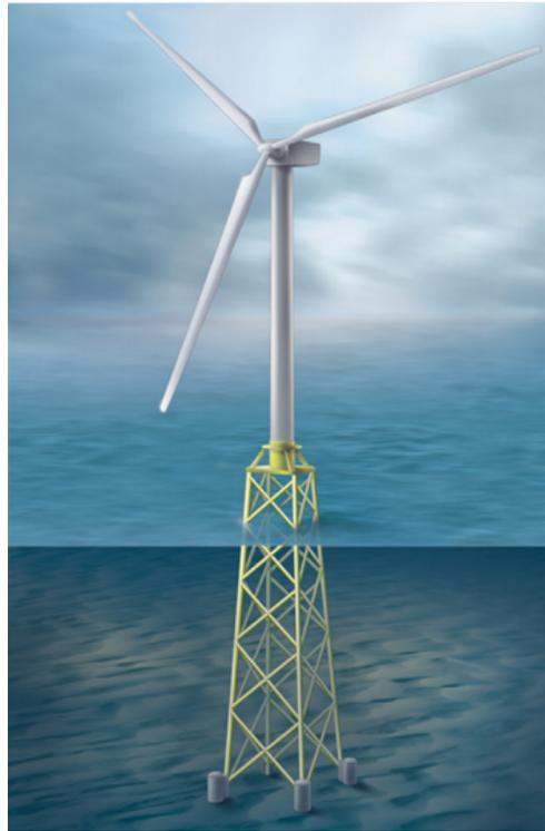
Figure 1.1: Wind turbine with steel jacket support structure [Dong et al., 2012].
