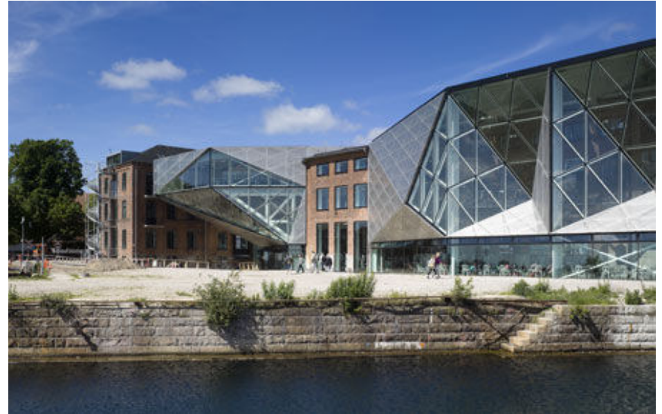
Fig. 31a. Illustration of covering up the existing façade when renovating, Kulturværftet in Helsingør
