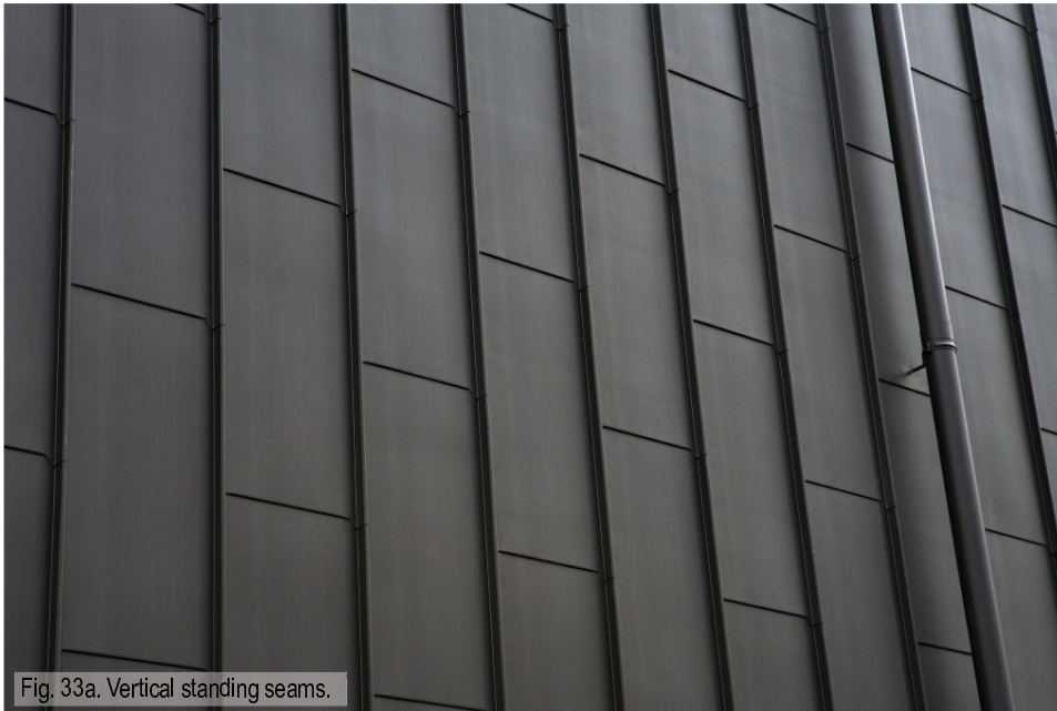
Fig. 33b. The standing seam gives a vertical expression to the facade.
