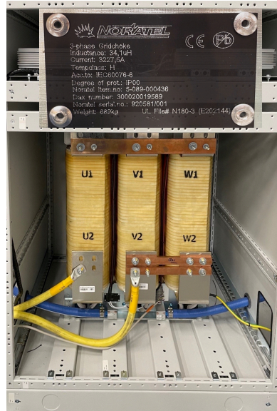
Figure 6.4: Load Inductor with Name Plate Details
