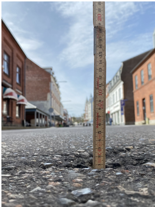
Figure 2.5. Picture from Holsteinsgade where a hole in the traffic lane is measured.
