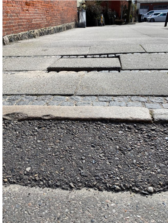
Figure 5.10. Picture from Holsteinsgade showing a defective part of the footway surface.
