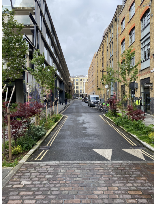
Figure 4.28. Picture from Shoreditch of a narrowed carriageway, which also works to reducing speed, with plantings at the sides.
