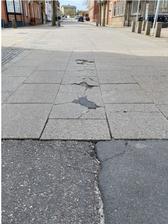
Figure 5.9. Picture from Holsteinsgade showing an uneven and defective part of the carriageway.
