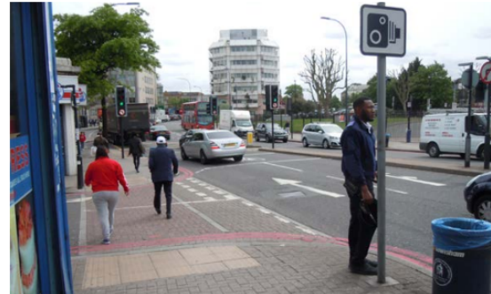
Figure 4.6. Example of raising and narrowing the carriageway side road aiming to make it easier and safer to cross (Transport For London, n.d.).
