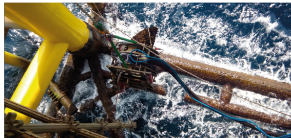
Figure 1.3: Crawler operating on the spider deck in the splash zone
