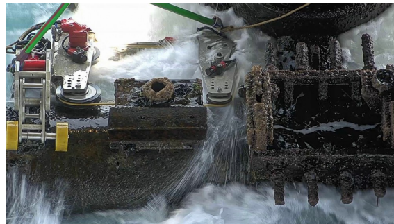
Figure 1.5: Crawler operating on offshore member with marine growth
