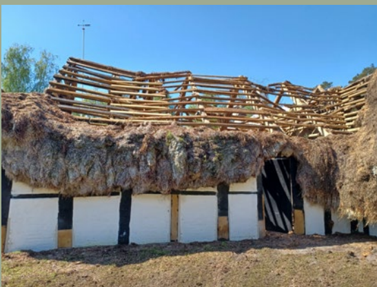
Illu. 16. Photographies of roof construction of original Læsø eelgrass houses. Photographies provided by Læsø Museum.
