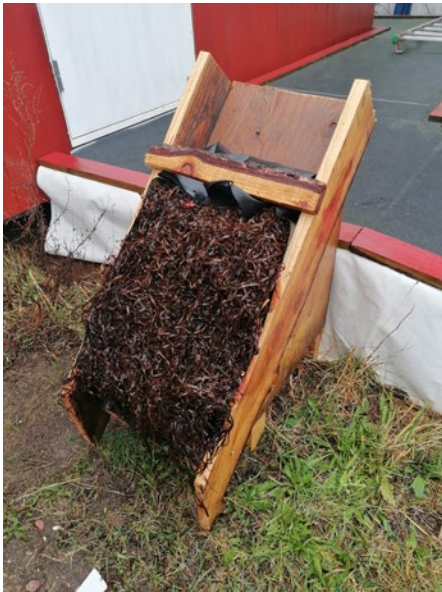
Illu. 157. Eelgrass roof construction for tiny house
