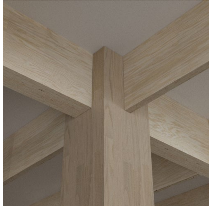
illu 106. LVL beam and glulam column joint
