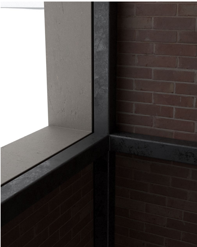
illu 85. steel frames within clay brick exterior
