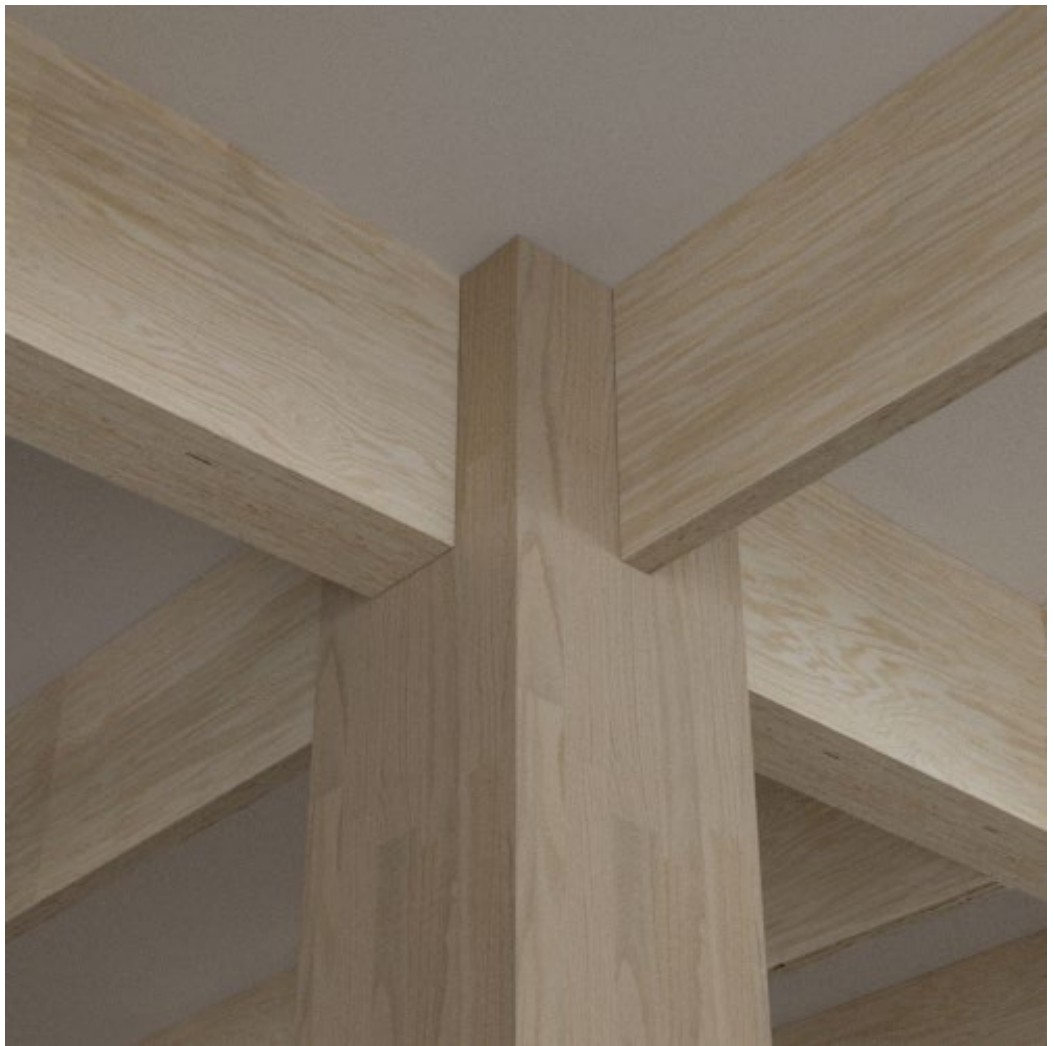
illu 47. beam-column connection
