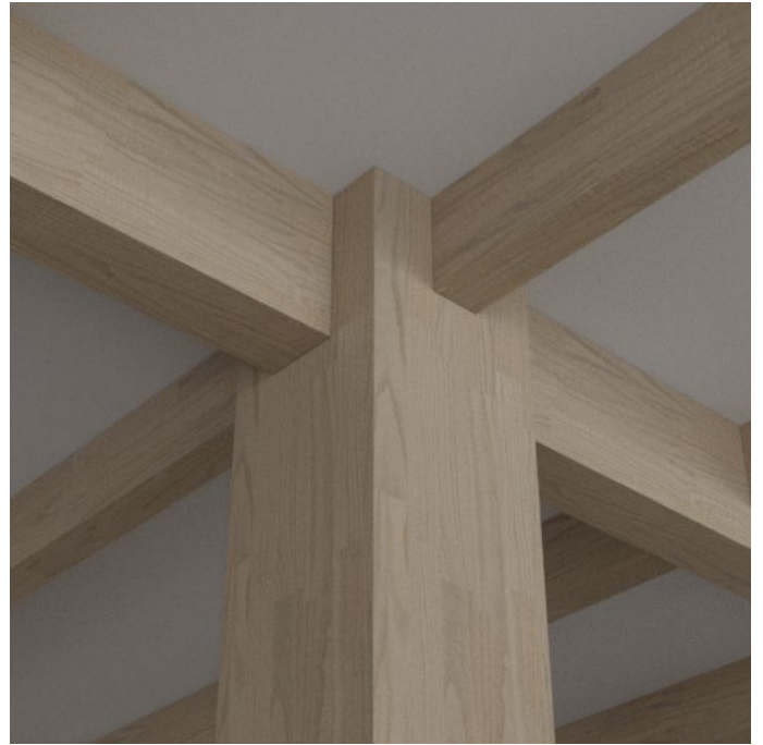
illu 105. glulam beam and column joint
