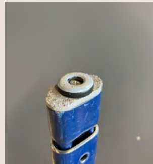
illu. 66: Slider shoe and a vibration absorber
