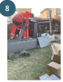
Before the electrician can take out the fuses, he measures the voltage to ensure the power is off.
