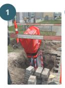
The barrier is removed so the electrician can access the damaged cabinet.
