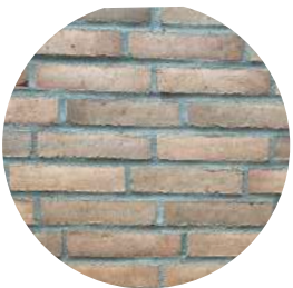
Illustration 38: Own photo Reused Red bricks
