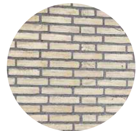
Illustration 40: Own photo Reused yellow bricks
