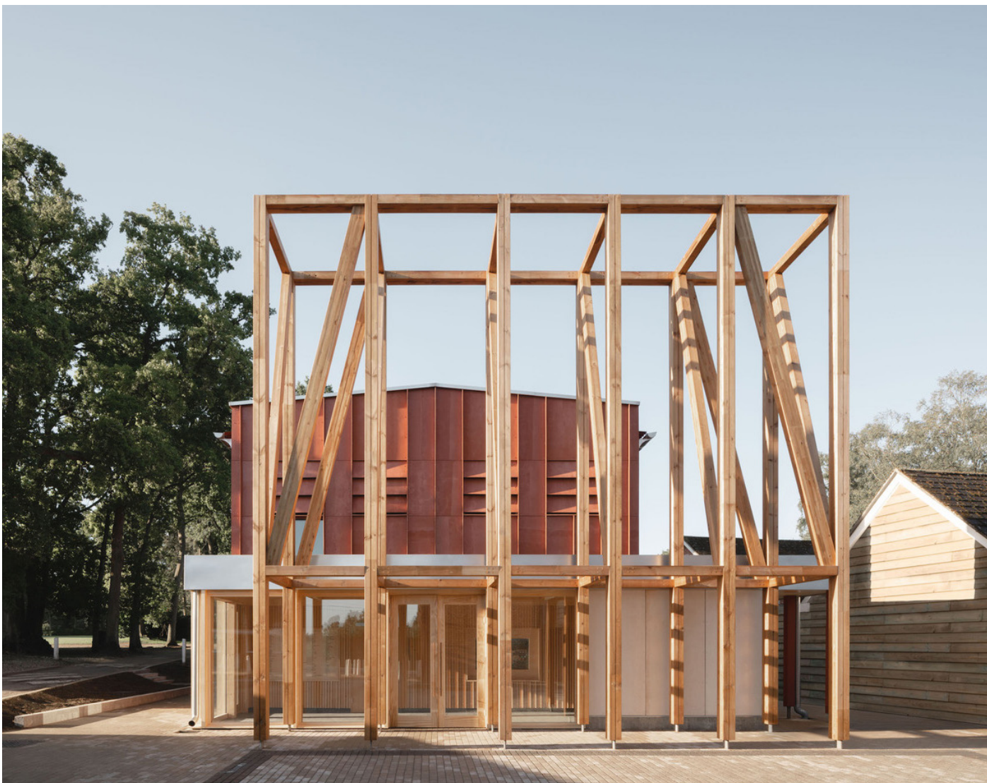
ill. 18: Picture of David Brownlow Theatre, Main entrance. Transitions.
