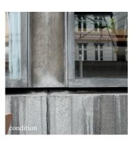
There is algaes on the concrete elements and the concrete is eroded and with visible reinforcement
