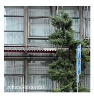
The principle of the modular system enables a free facade; there is no need for stabilizing, so apart from the load-bearing columns, it can consist of lightweight elements. This underpins the open/free facade which is characteristic of modernist architectural principles and was also a highlighted quality in the design of the "Fynsplanen" as it allowed facade freedom
