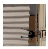
The asbestos-cement panels are corrugated.
