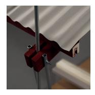
The junction is simple: all elements meet in a bolted connection.
