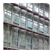
The existing system consists of: steel pipes, painted wood profiles, asbestos-cement roof, bolt connections.
