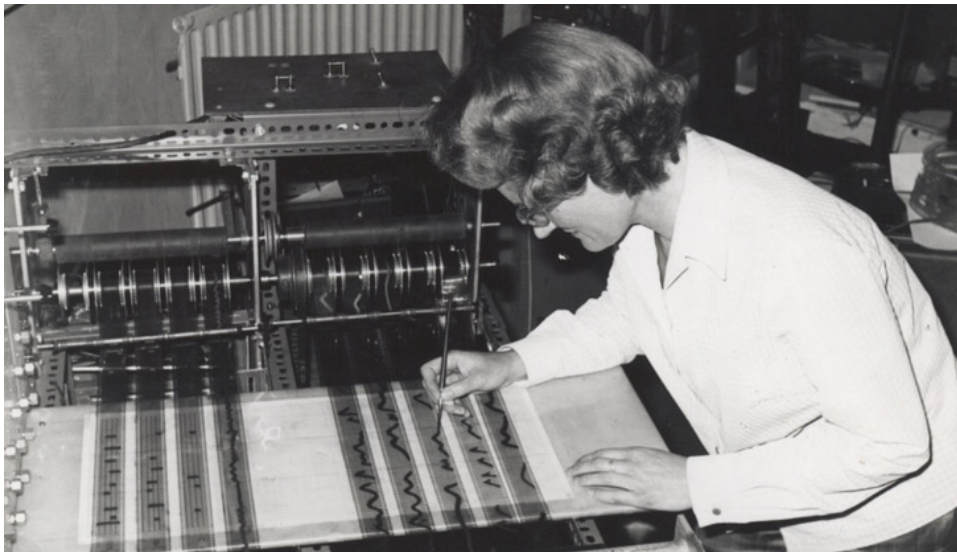
Figur 2.2: Promotional photo from around 1966, Oram is depicted working on the analogue volume control section. To the left of the film tracks, there are three digital pitch control tracks followed by the vibrato track. 2
