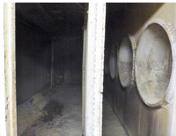
Figure 4.3: The five ventilation holes to the right leading the polluted air from the pigsty and into the test facility and to the left the first biofilter.
