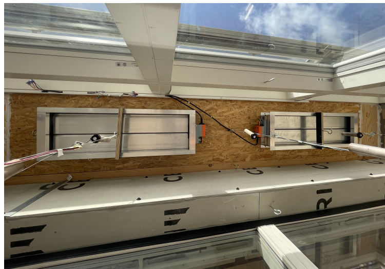
Figure 3.13: The separation between the DSF cavity and plenum box is closed during the cooling mode.
