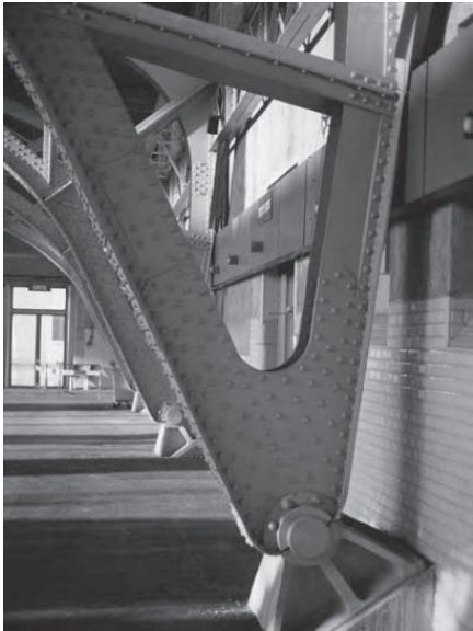
Fig.32. (top) The global form of the original slaughter hall in Lyon (1914) is a three-hinged frame in steel.
