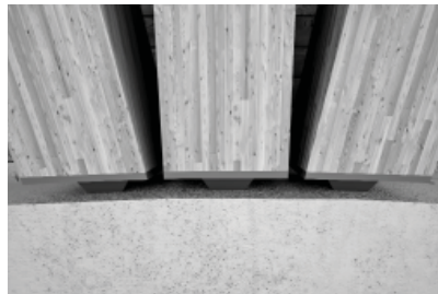
II - CLOSE UP OF THE JOINT BETWEEN THE ARCHES AND THE ARCH FOUNDATION
