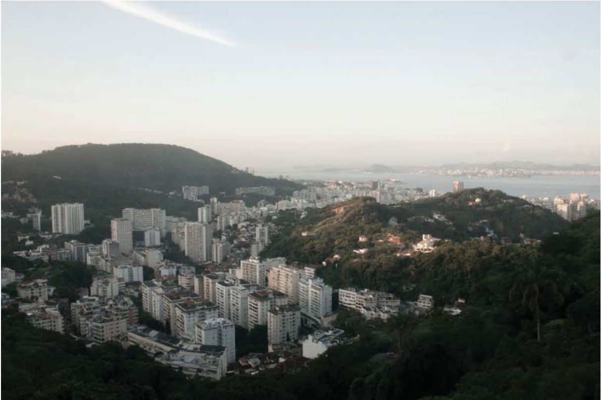
ill. 33 View North - towards Centro
