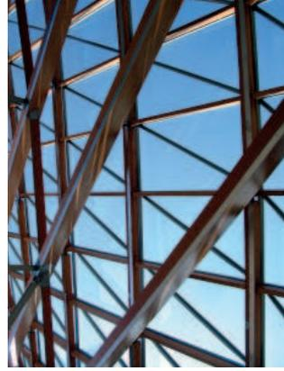
*Glulam beams is used as the main structure and to carry the floors. The facade will consist of glass.*
