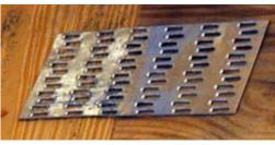
Example of metal plate connector used to connect two coplanar wooden elements.
