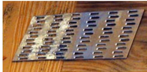
Example of metal plate connector used to connect two coplanar wooden elements.
