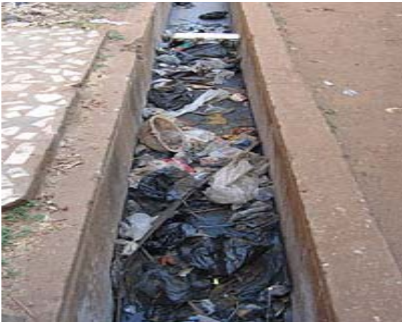
Fig.1.3: Waste blocking drain
