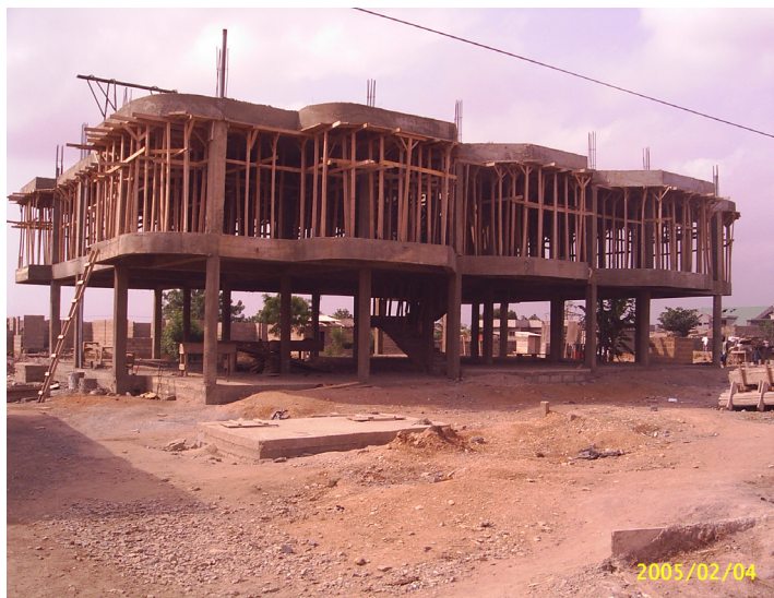
Fig 6.2: picture of a timber been used as formwork. Date: 04-02-2005
