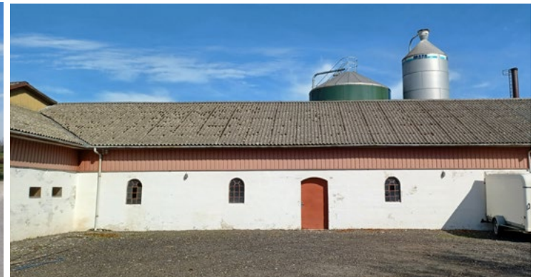
Illu. 188 - Lime washed brick facade with a metal plate bond on the top of the facade.
