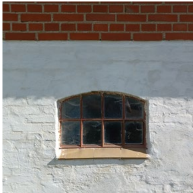
Illu. 186 - Characteristic, horizontally oblong cast iron windows with mullions and a rounded top.
