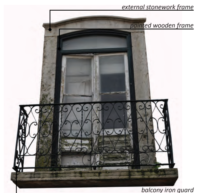
ill. 040_ ensemble of window, frame, external frame and iron guard
