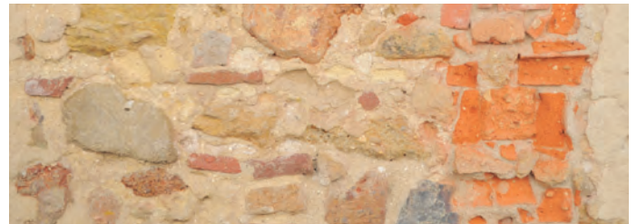
ill. 034_ detail from an external wall, lime and sand mortar
