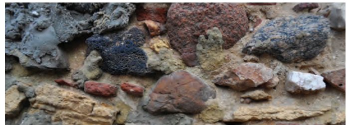
ill. 033_ detail from an external wall, lime and sand mortar
