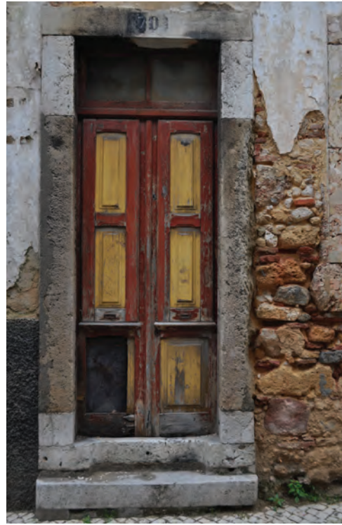
ill. 032_ facade in decay, where the structural wall can be seen, made of lime and sand mortar
