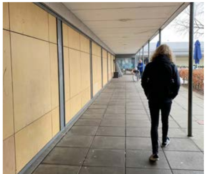
III.45 | View of Rema 1000's facade. Sundparken, Horsens.
