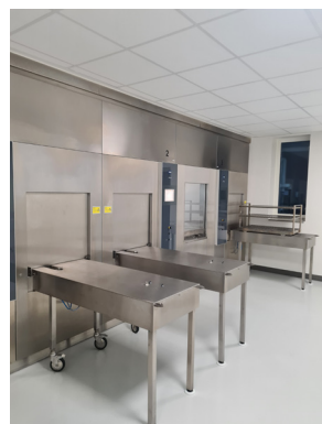
III. 22. Lock to the sterile zone through the steam autoclave
