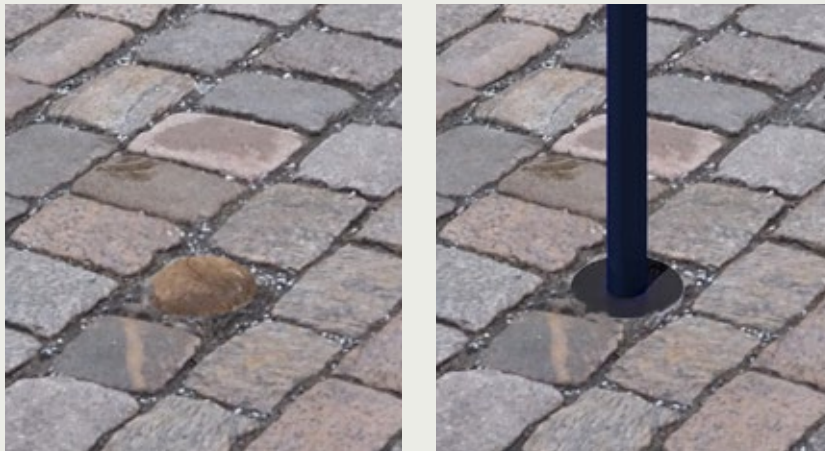
Illustration 101. Paving detail, showing the base for tent post - not used and used.
