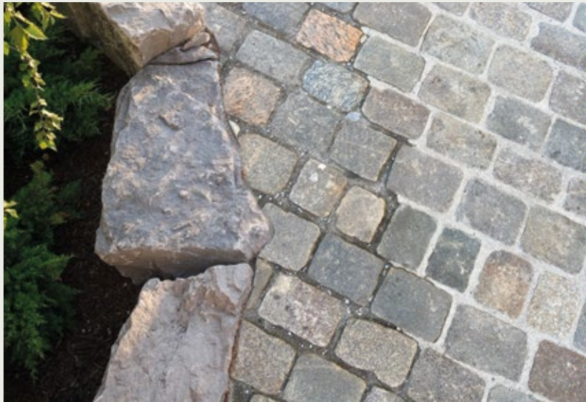
Illustration 121. Paving detail along the edge of the rain gardens
