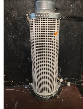
**Figure 1.3** Inlet diffuser for displacement ventilation
