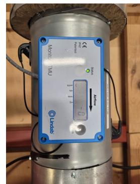
**Figure 1.5** Flow meter used for both return and AHU.
