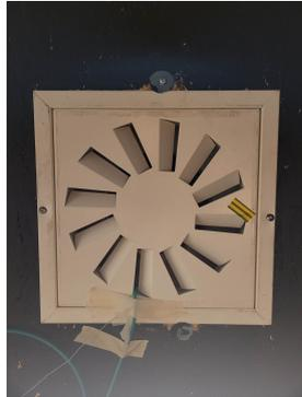
**Figure 1.2** Inlet diffuser for mixing ventilation
