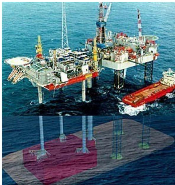
**Figure 1-1: The production platform, Siri, and a rig (to the right) to drill the wells. The platform is founded on three legs (steel tubes) entering the caisson (the red box) on the seabed. The legs were partially grouted in 2003 as reinforcement of the legs due to change in the design loads.**
