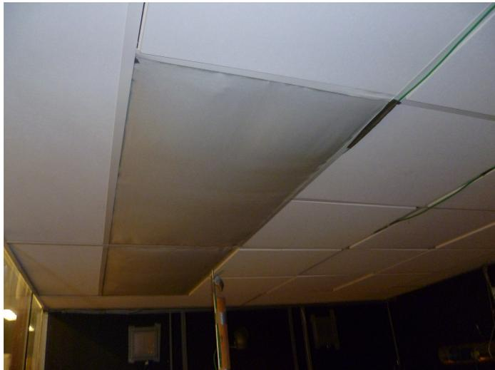
Figure D.1: The inlet diffuser mounted in the ceiling.
