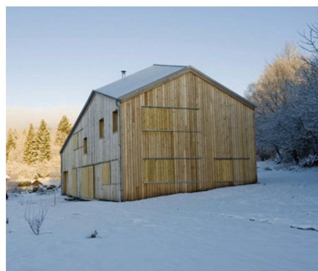
Ill 07. The wooden shutters lower the heatloss from windows during the night.
