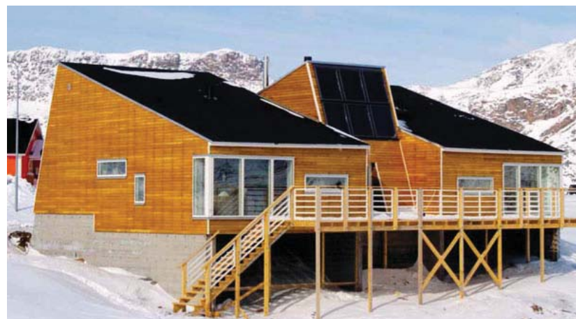
Ill 33, The lowenergy house in Sisimiut, ARTEK, DTU. The consumes 140 kWh/m 2
