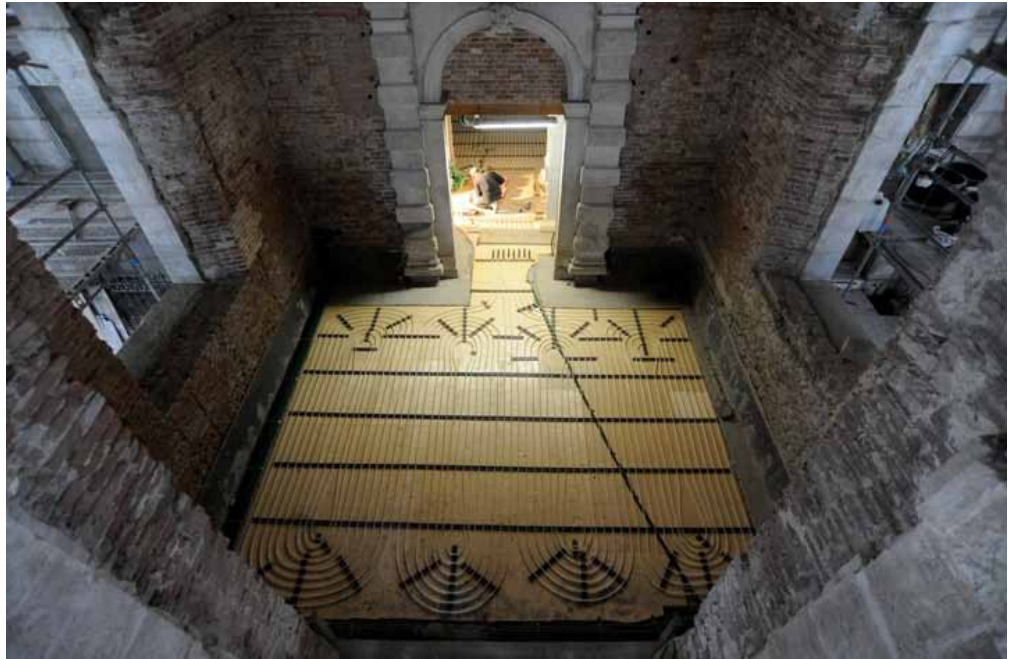
#18 Installation of floor heating in Tadao Ando's restoration of Punta della Dogana, Venice
