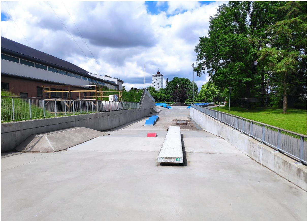
Figure 9: Skate Park with detention basin function in Gladsaxe sportscenter (own Figure by author)
