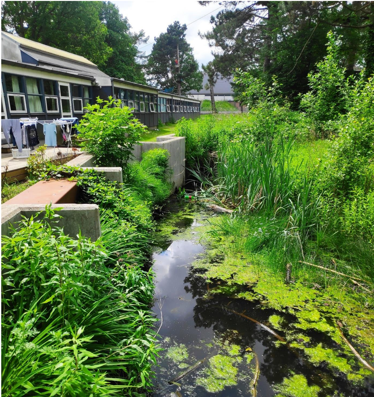
Figure 11: Retention Basin in Gladsaxe sportscenter (own Figure by author)
