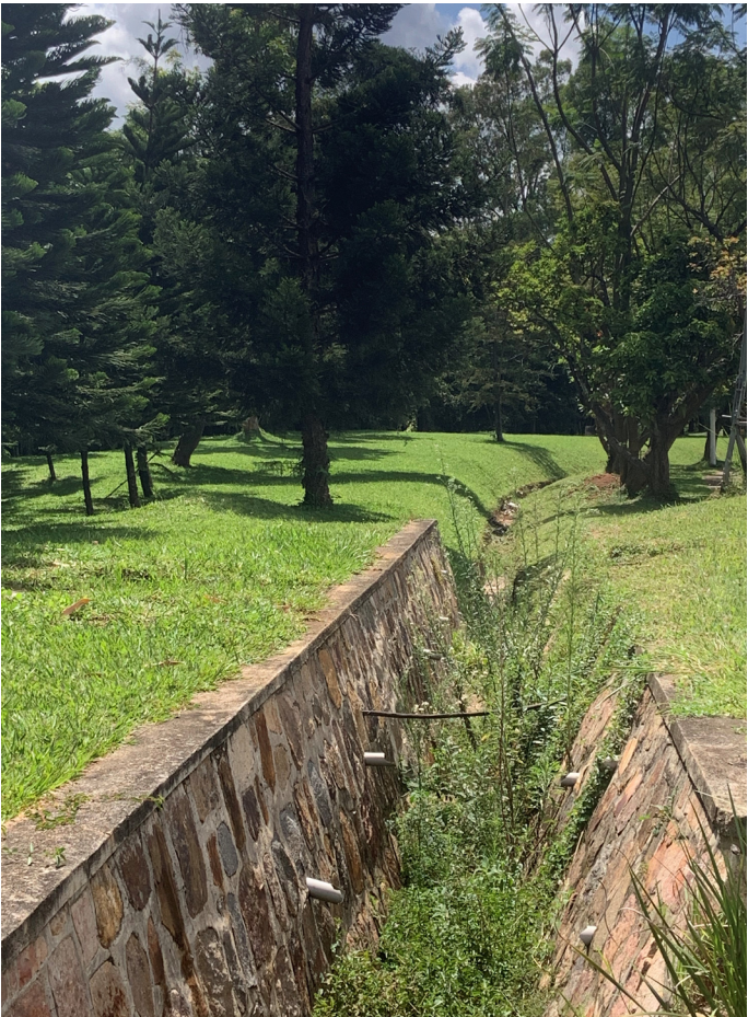
Image 34. Green Drainage Channel, Example 2
