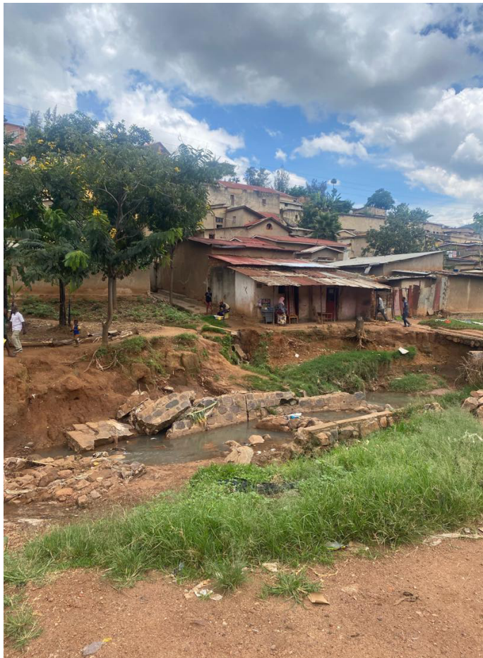
Image 18. Collapsed River Channel in an Informal Settlement in Katabaro
