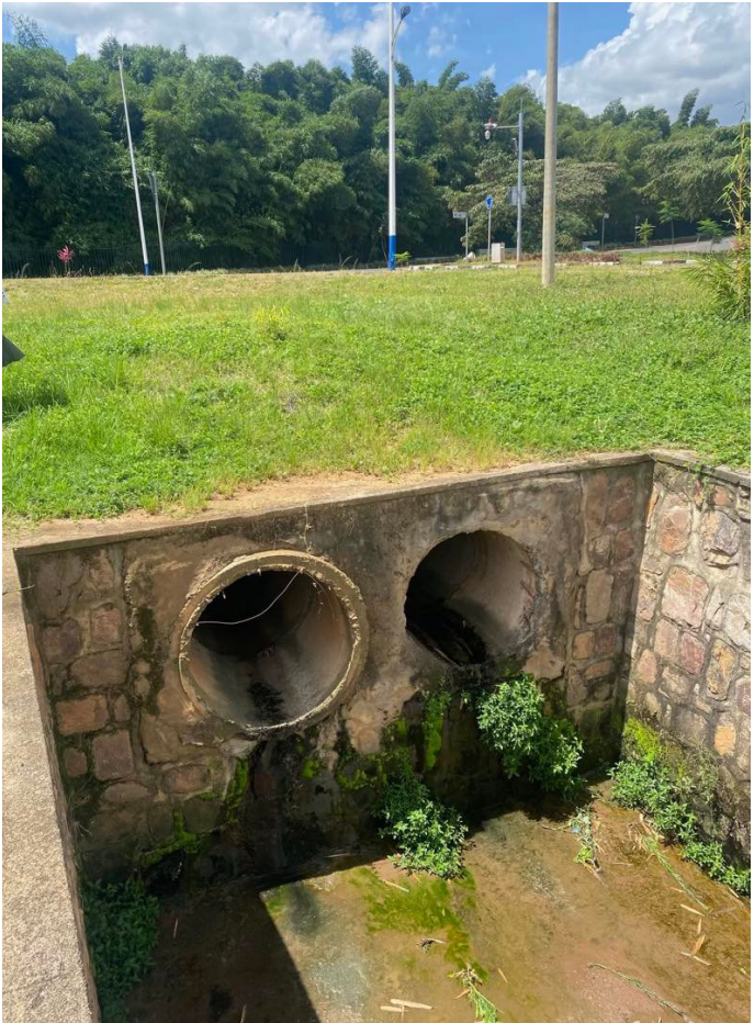
Image 11. Closed Underground Drainage System
