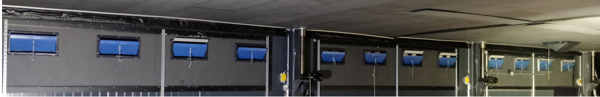
Figure 2.5: Image of the placement of the DA 1211 air inlets inside the air physical laboratory.
