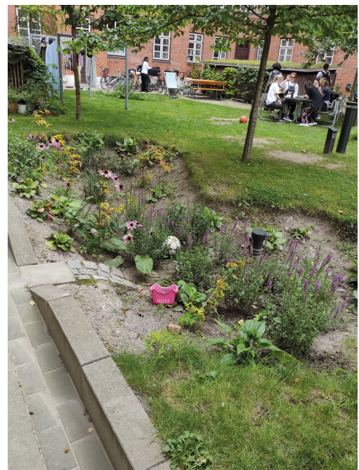
Figure 3: Rain garden, fed with roof runoff (own figure).
