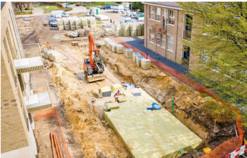
Figure 4: Rockflow installation in an urban area (ROCKWOOL, n.d.).
