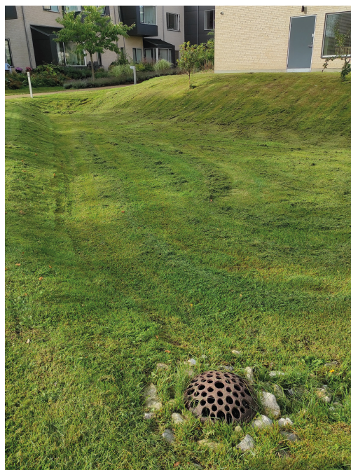
Figure 2: Infiltration ditch, fed with roof runoff (own figure).
