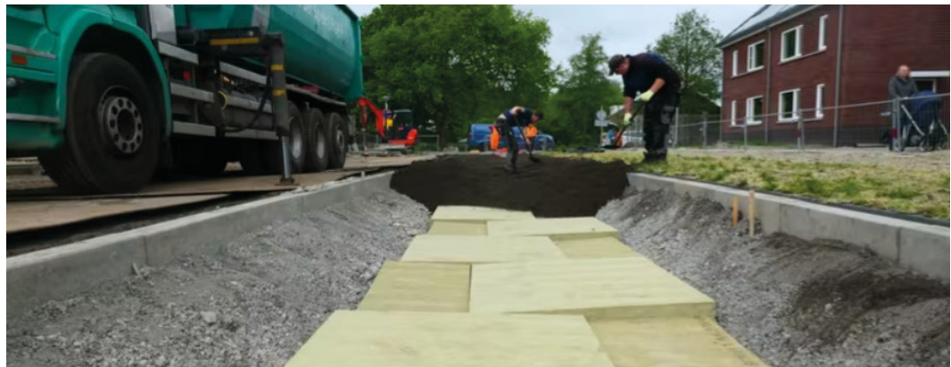
Figure 29: Installation of Rockflow in combination with a bioswale in Zoeterwoude (ROCKWOOL, n.d.-b).
