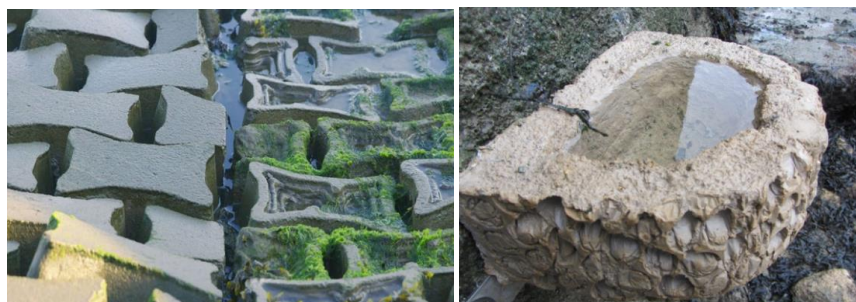
Concrete blocks and rock pools in sea walls (EConcrete & Marineff in Quintana et al., 2021, p. 15).
