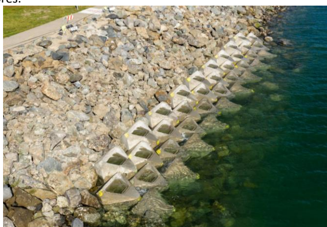
The project, "Coastalock" provide coastal defense while simultaneously providing habitats for marine organisms to colonize it, San Diego Bay, US (Crook, 2021).
