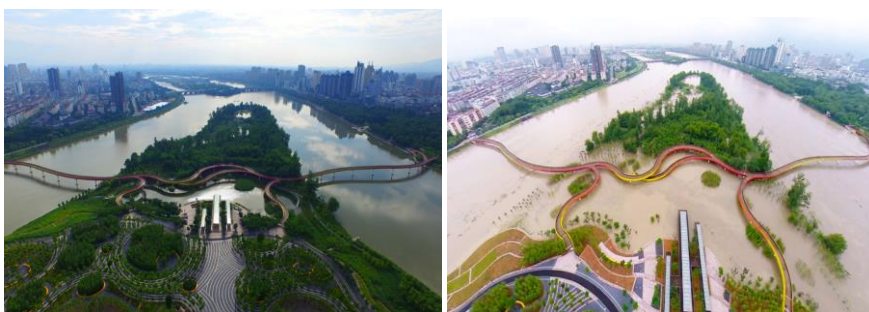
The realized project Yanweizhou were previously dominated by a concrete wall criticized to destroy the natural ecosystems. Now the area constitutes terraced ecological embankments allowed to flood. Yanweizhou Park in Jinhua, China. The left photo is at an average water level and the right photo is during a flood (Hobson, 2015).
