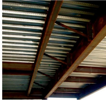
**Figure 6.7:** Diagonal 'kicker' braces [Hamburger and Malley, 2016]
