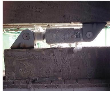
**Figure 4.6:** Fluid viscous damper employed on a structure. Photo courtesy of roadjz.com.
