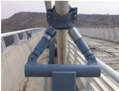
**Figure 4.5:** Fluid viscous damper employed on a bridge. Photo courtesy of roadjz.com.
