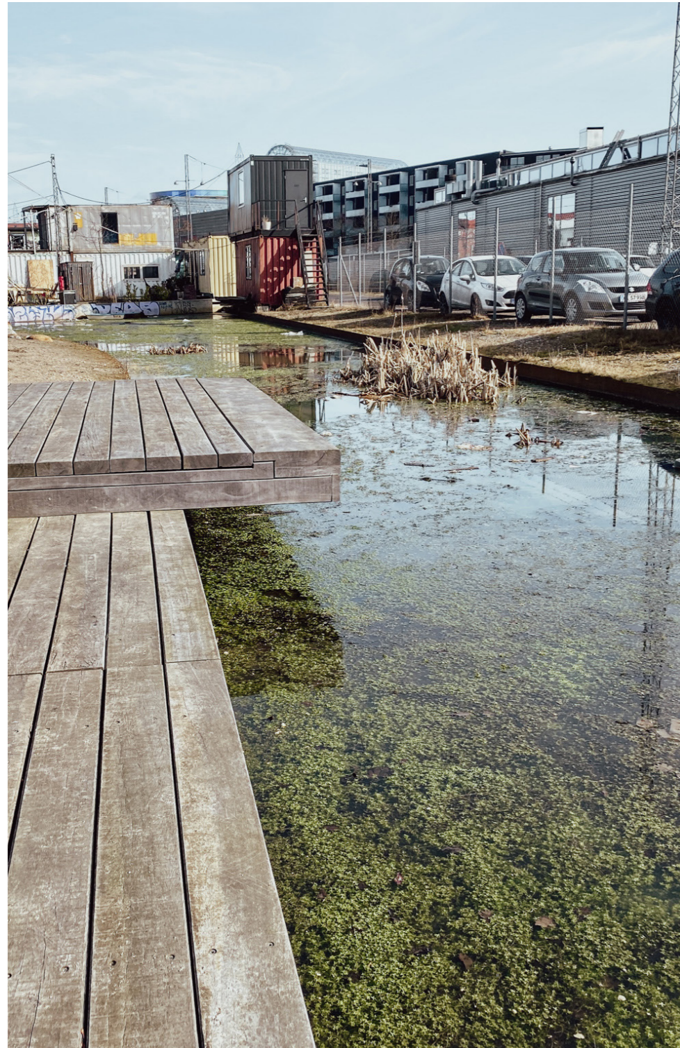
Ill. 32 The neglected retention pond
