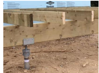
Figure 40 Floor deck illustration. Wood joist on screw pile foundation. (Goliath Tech )
